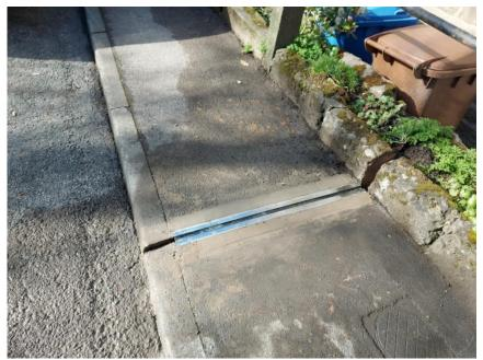
Figure 6-1 - An example of a cable tray installed into the footpath
